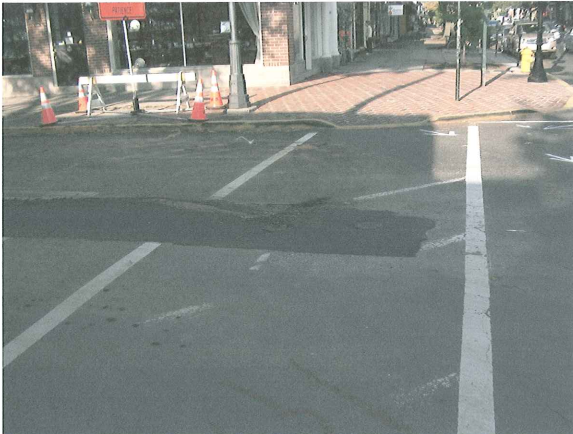
View of New Water Main Location at Kings Highway East
