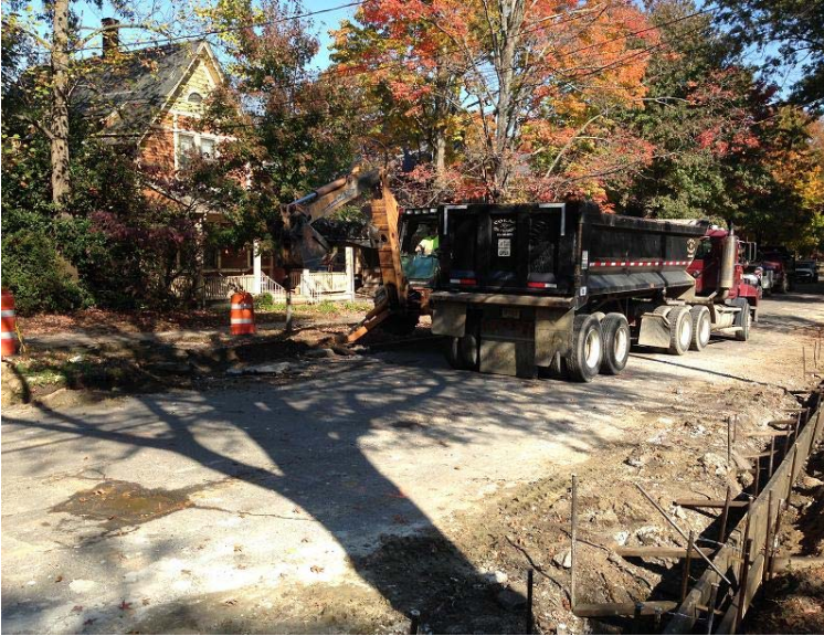
Removal of Curb Between West End and Estaugh Avenues
