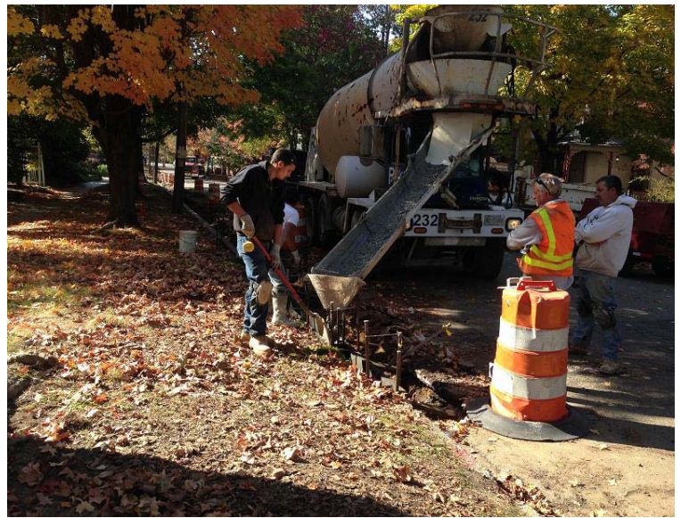
Pouring New Curb Between West End and Estaugh Avenues
