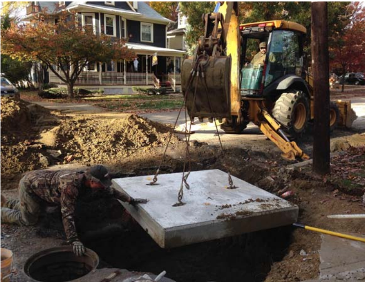
Installation of Inlet Base Slab at Estaugh Avenue
