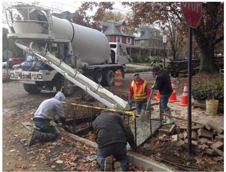
Pouring Concrete Curb Ramp at Westmont Avenue
