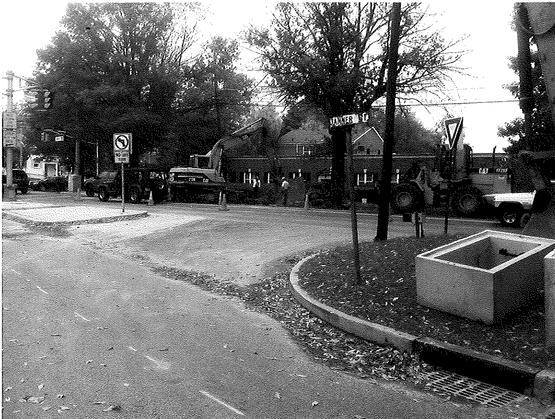
View of the Installation of the New 48 Inch Diameter Storm Sewer in Haddon Avenue
