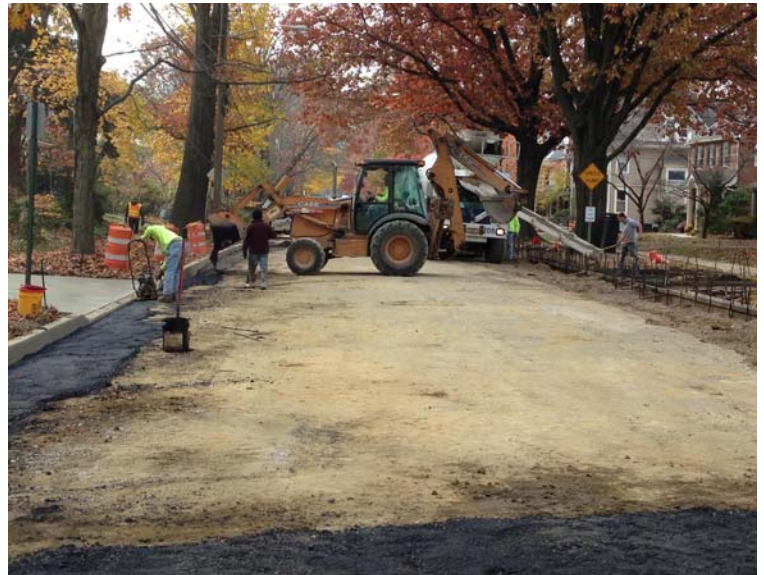
Installing New Curb and Driveway Aprons Between Linden and Estaugh Avenues
