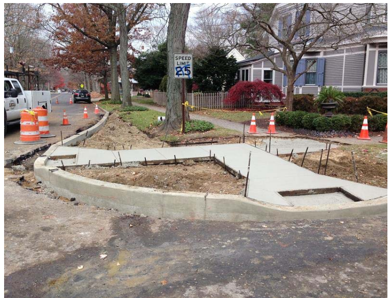
New "Bump Out" Realignment at Northwest Corner of West End Avenue
