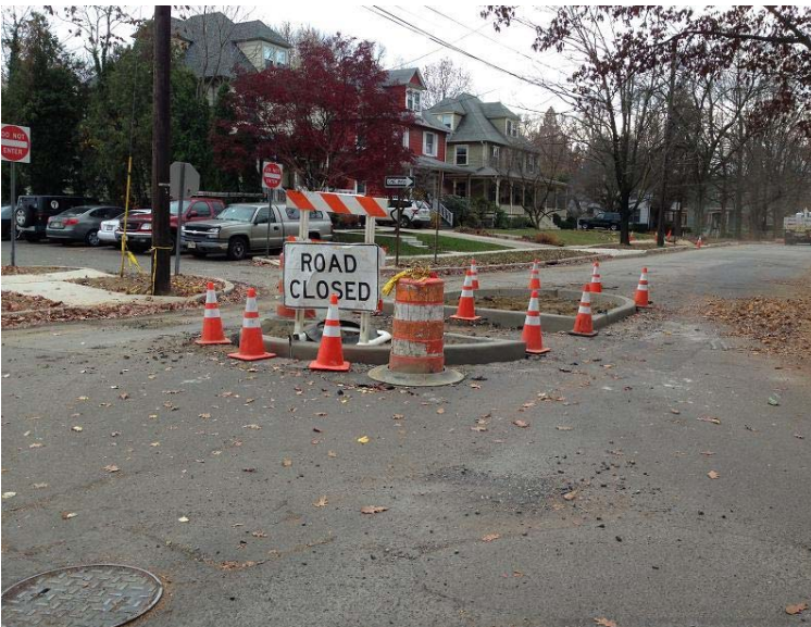
New Median Island at Westmont Avenue
