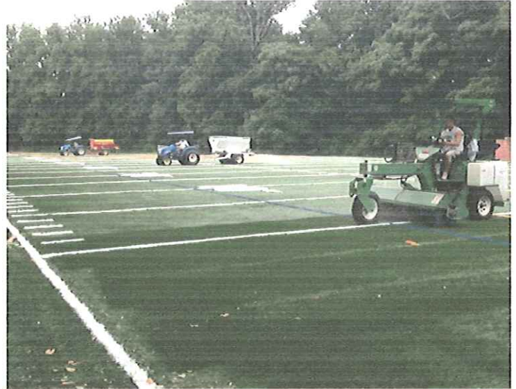
Anniversary Field ~ Installation of Infill
