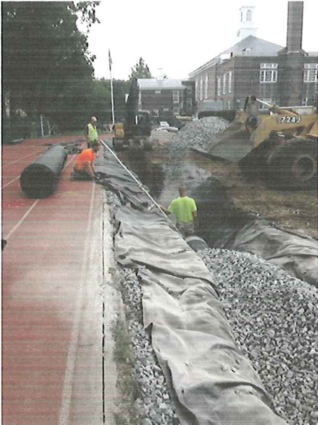
Stadium Field ~ Installation of Perimeter Drain Pipe
