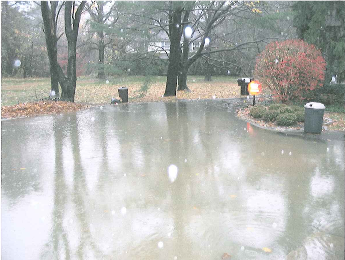
View of the Drainage Issue at the End of Lane of Acres
