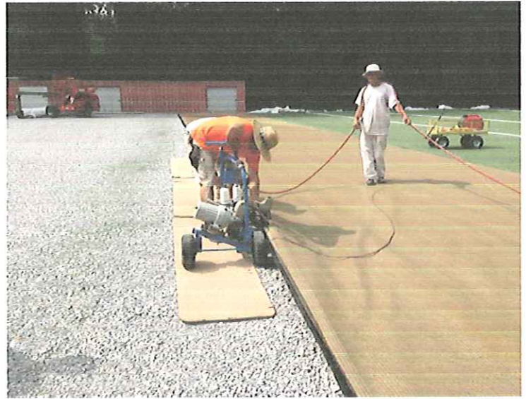
Anniversary Field ~ Stitching Together Sections of Turf
