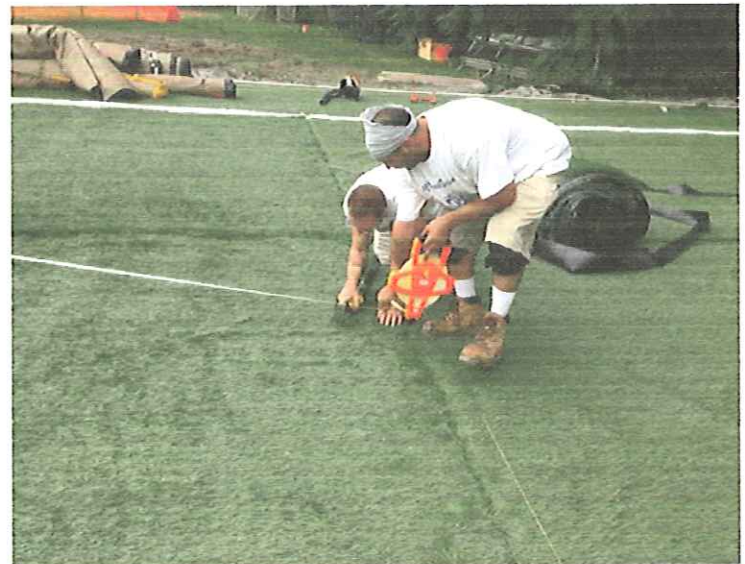
Anniversary Field ~ Cutting for Installation of Team Lines
