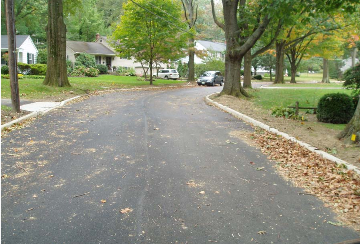
View of the New Paving Along Pennbrook Drive
