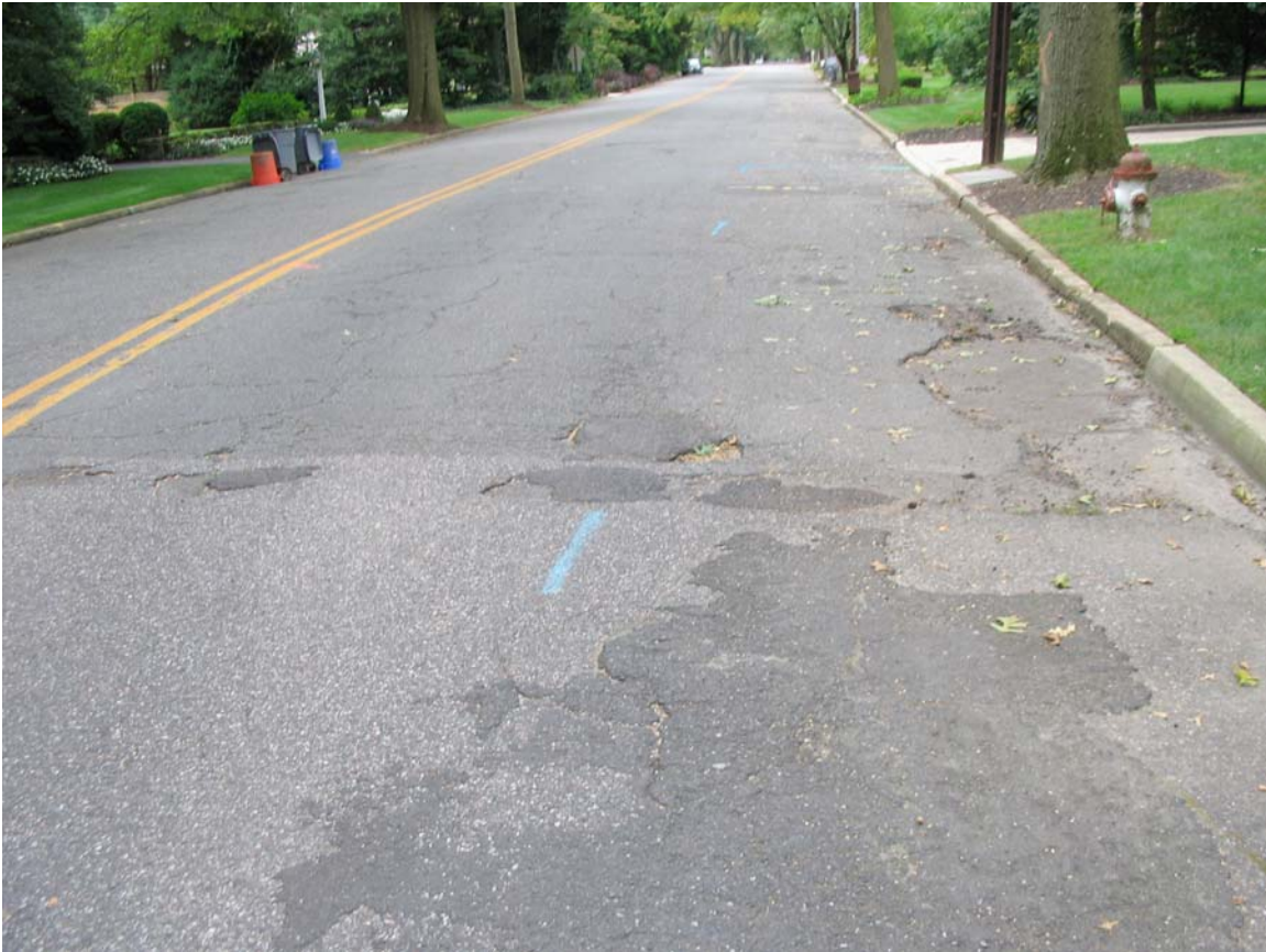
View of Old Fire Hydrant to be Replaced
