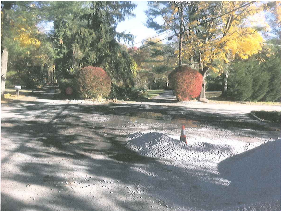
View of the Cul-de-Sac Area Prior to Repaving the Roadway
