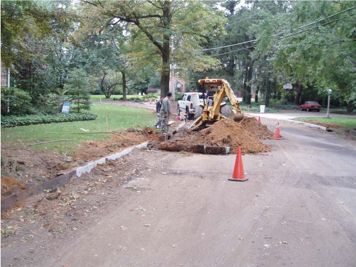
View of Stormwater Inlet Repairs
