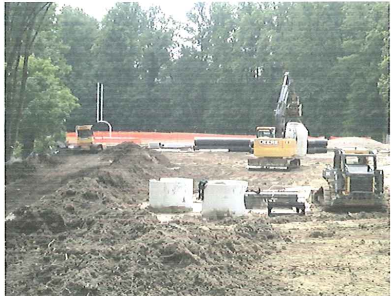
Grading of Anniversary Field and Delivery of Materials
