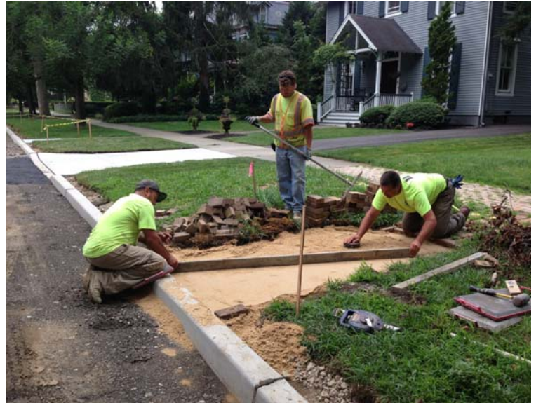
Resetting Brick Service Walk at 212 Washington Avenue
