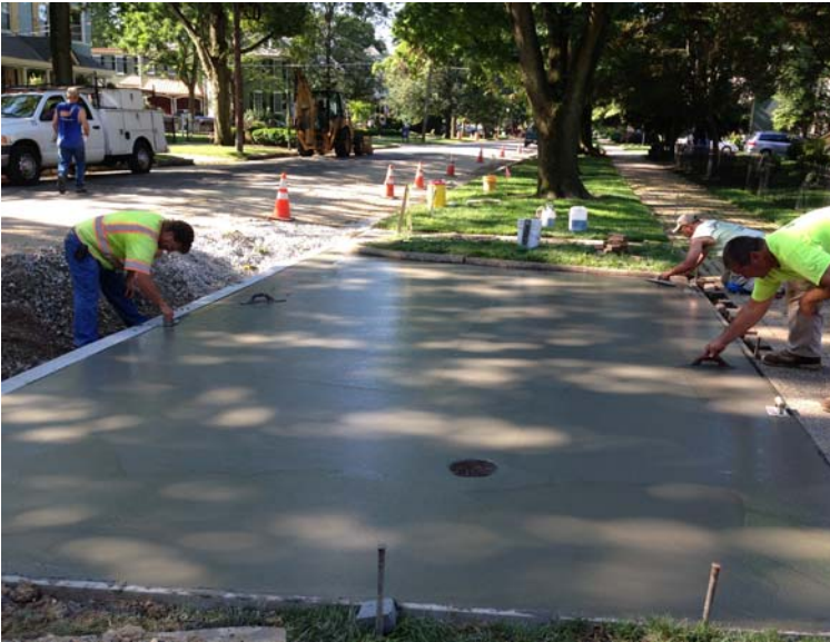
Finishing Driveway Apron at 228/232 Washington Avenue
