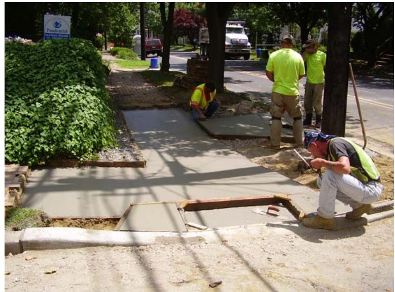
Installation of curb ramps at Potter Street/Springfield Terrace
