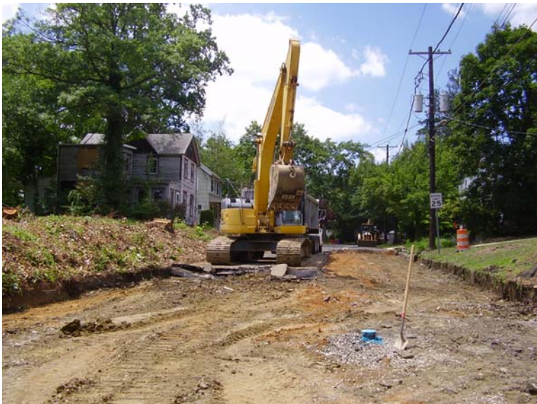
Removal of pavement on Potter Street
