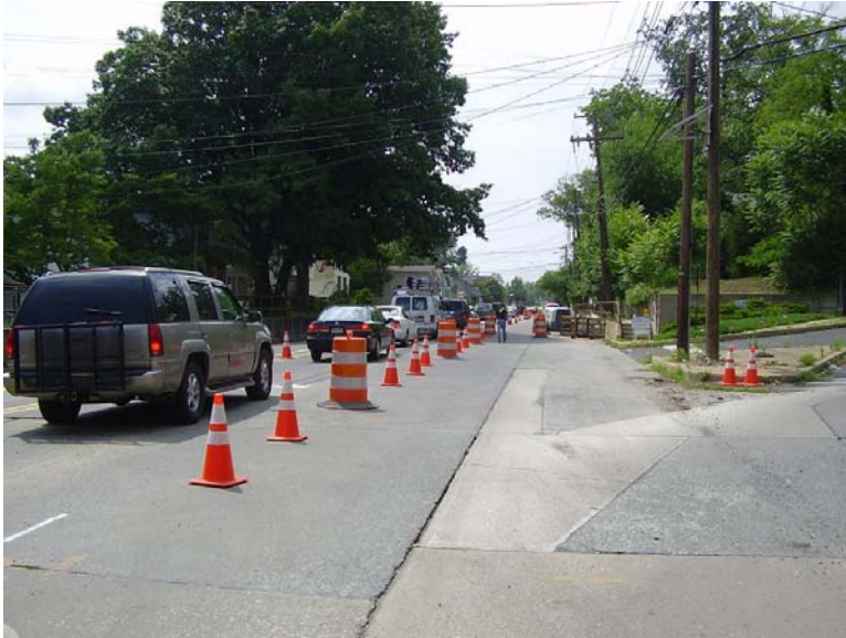
Traffic Control on Ellis Street
