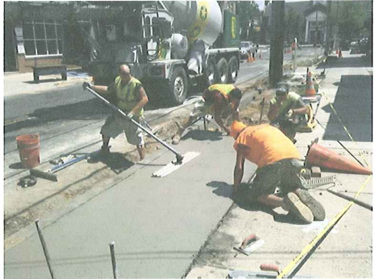
Driveway Apron Construction Along West Side of Road
