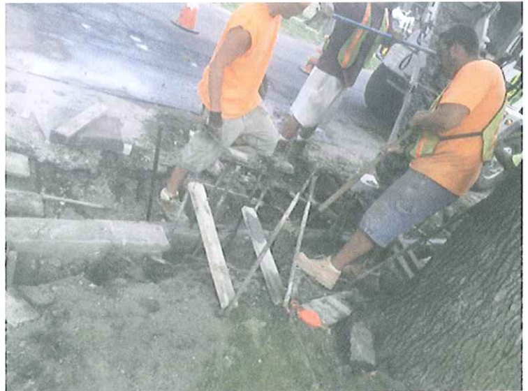
Slate Curb Resetting
