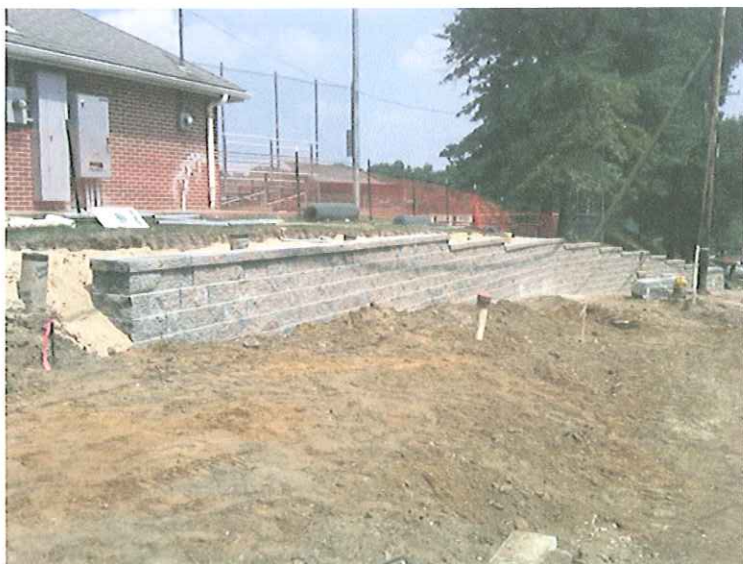
Completed Retaining Wall On Potter St. Adjacent to HLL Fields
