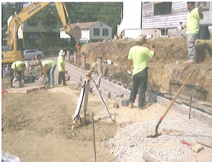
Retaining Wall Construction @ MacDonald Park
