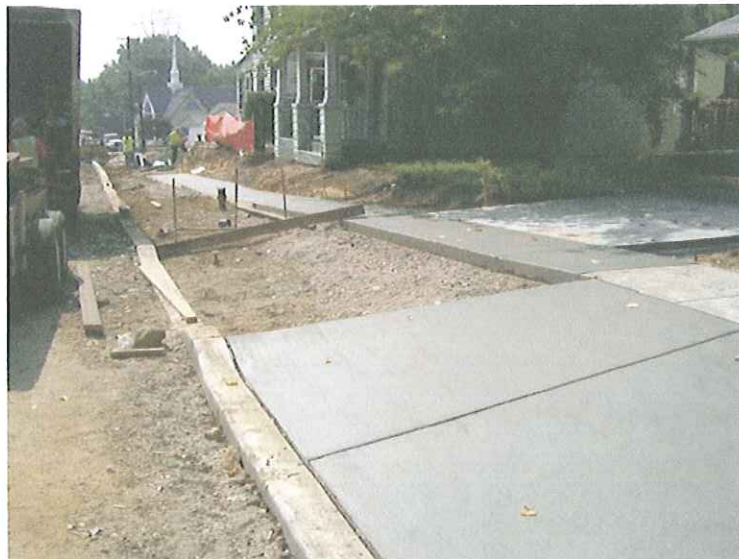
Driveway Apron & Sidewalk Construction On Potter Street
