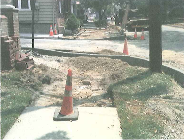
Curb & Sidewalk Construction At Clement Street
