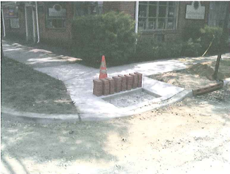
Partially Completed Curb Ramp At Wilkins Avenue
