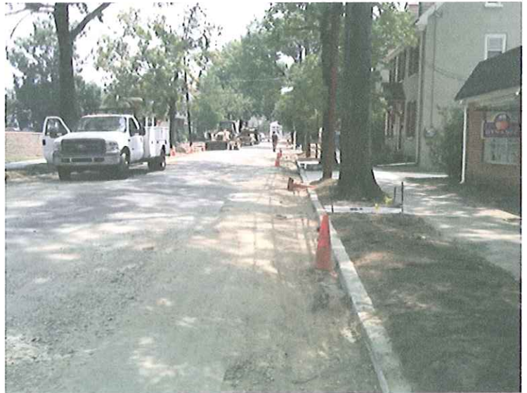
Completed Curb & Sidewalk Along West Side of Road
