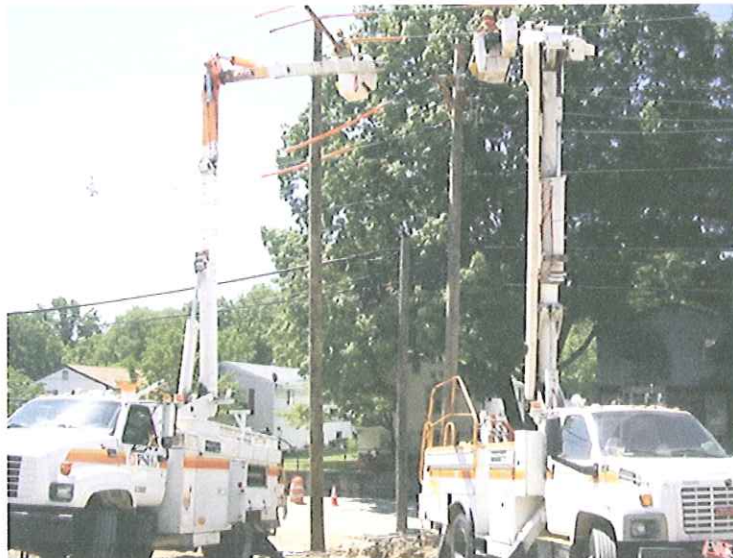
Utility Pole Relocation On Ellis Street
