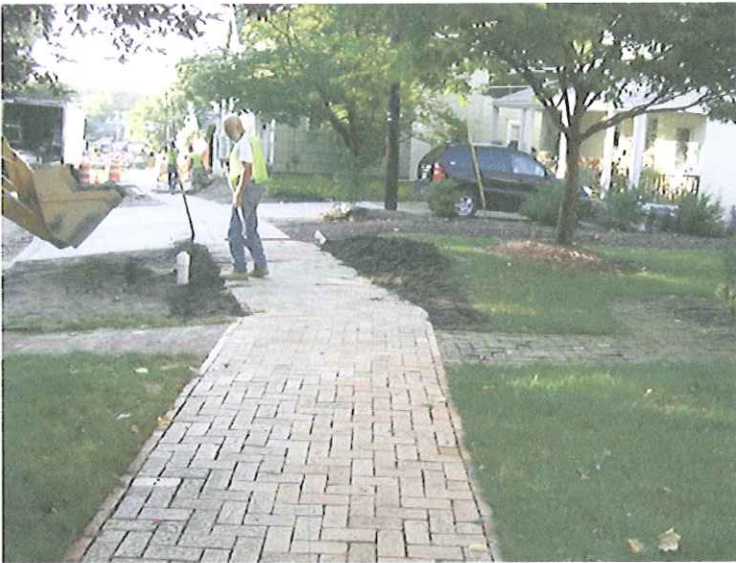
Completed Brick Walkway (re-set) On Potter Street
