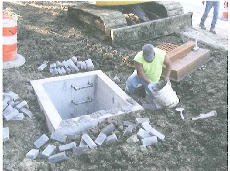
Stormwater Construction On Ellis Street Across From Lincoln Ave.
