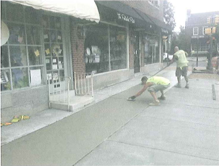
Sidewalk Construction At Kings Highway
