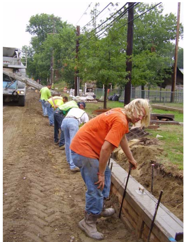
Curb construction on Ellis Street
