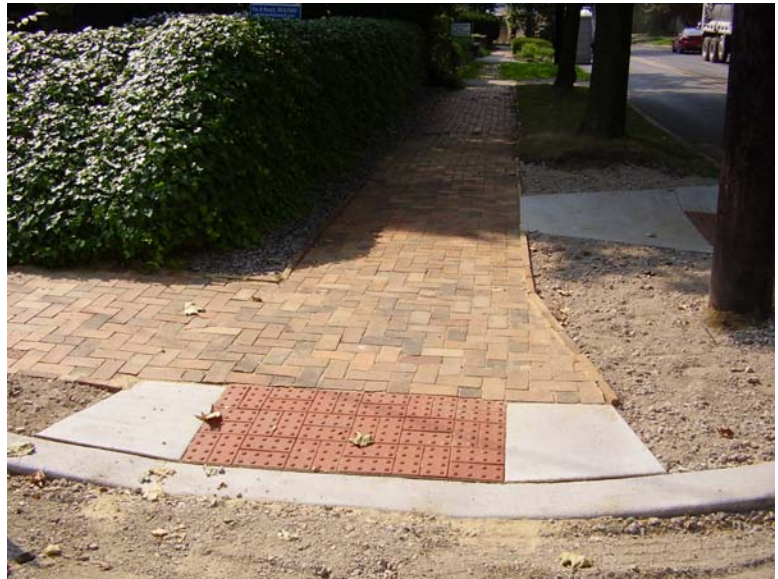
Completed ADA Curb Ramp at Springfield Terrace & Potter Street
