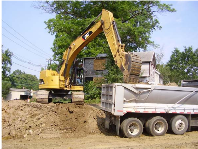
Excavation/Lowering of MacDonald Park
