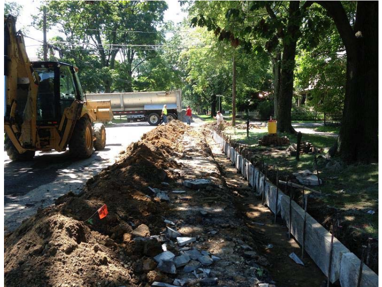
Resetting Slate Curb at 320 Washington Avenue
