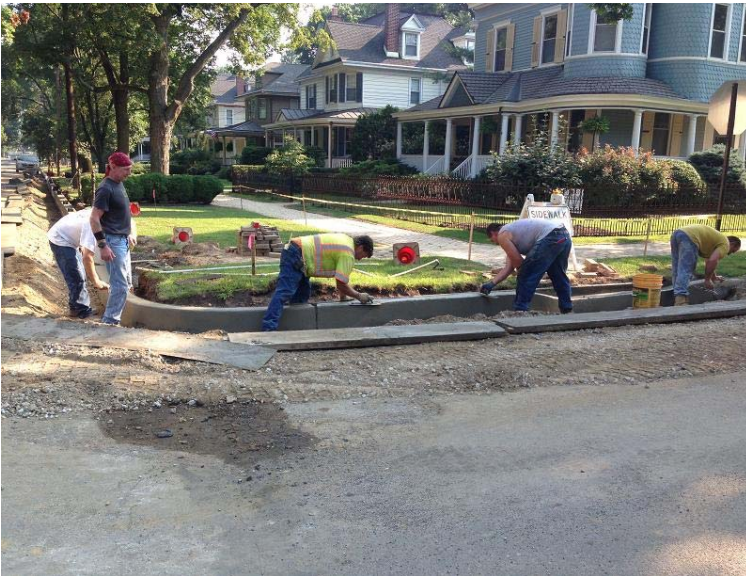
Finishing Concrete Curb on Washington @ W. Cottage Avenue
