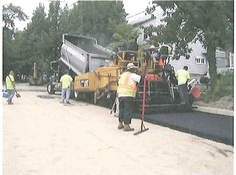
Base Paving on Potter Street.
