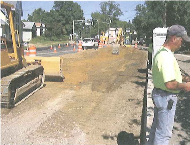
Grading for Base Course On Ellis Street
