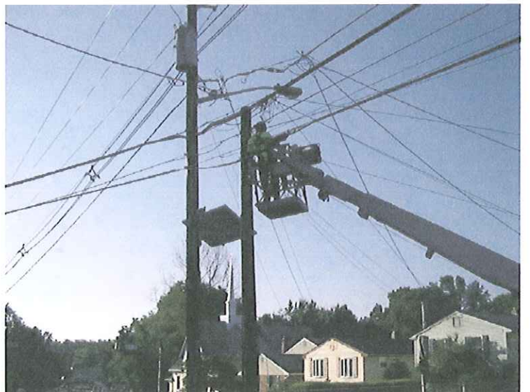
Relocation of Verizon Lines From Existing Pole at Potter Street
