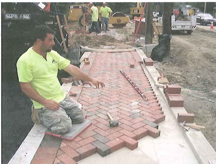
Construction of Brick Paver Crosswalk at Potter/Ellis Intersection
