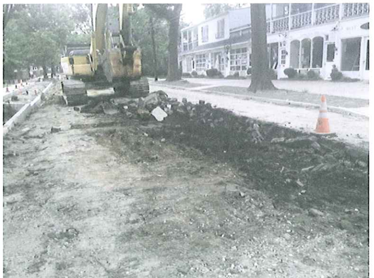
Roadway Excavation of Tanner Street
