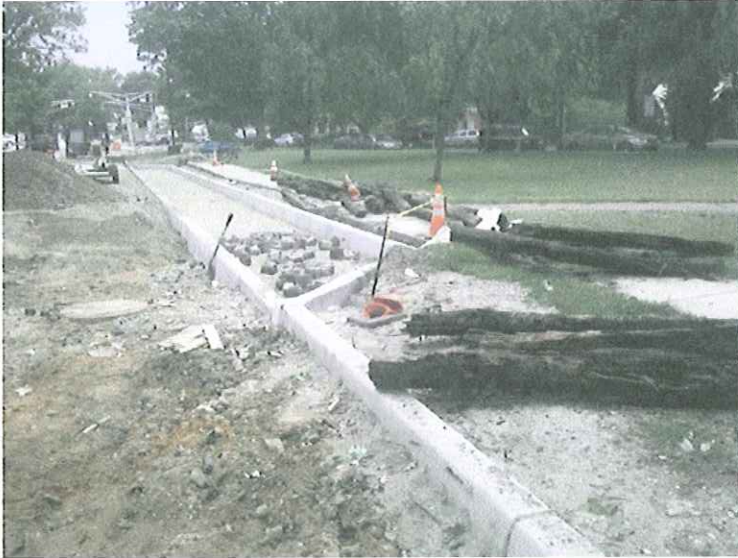
Expanded Parking Areas with Reclaimed Cobblestones & RR Ties
