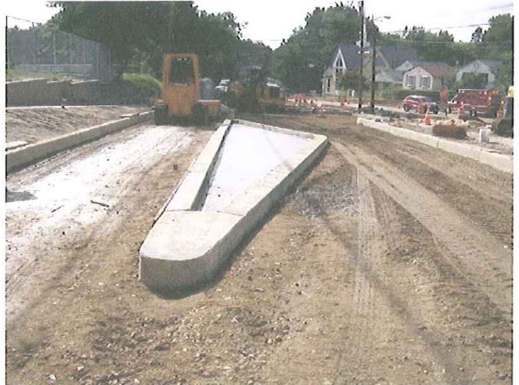
New Concrete Median on Potter Street.
