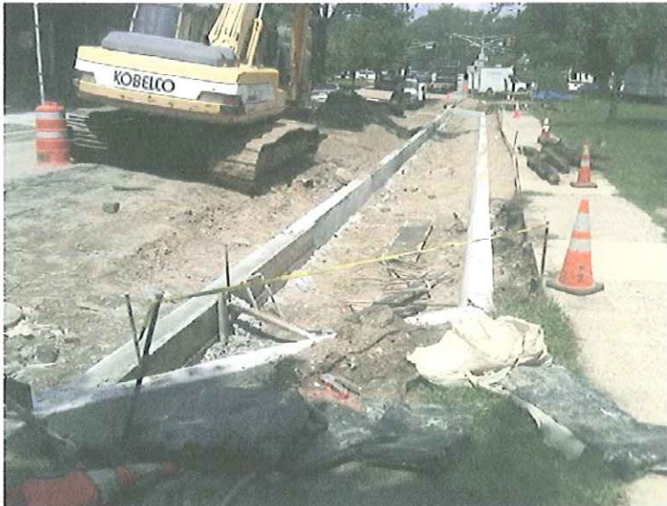
Curb Construction for Library Point Parking Areas
