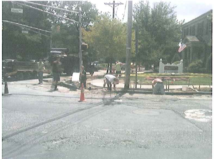
Curb Construction @ Southwest Corner of Euclid Avenue
