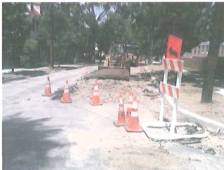
Roadway Excavation on Tanner Street @ Wilkins Avenue
