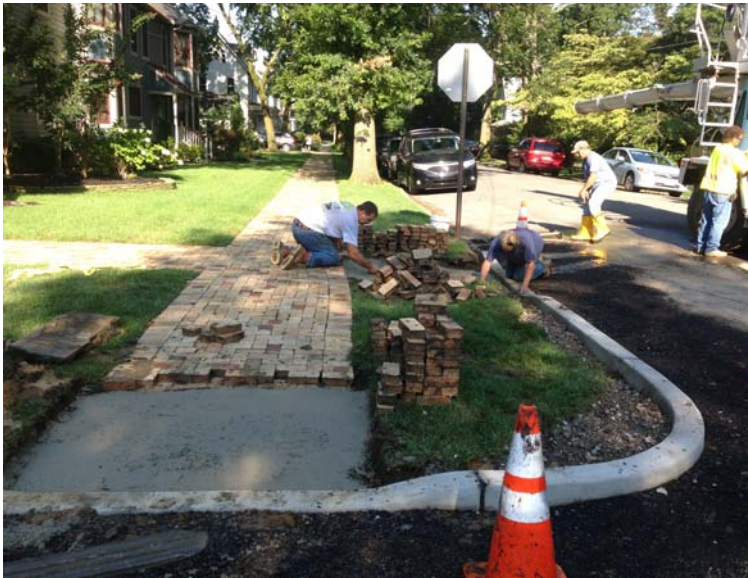
Resetting Brick Sidewalk on Washington @ W. Summit Avenue
