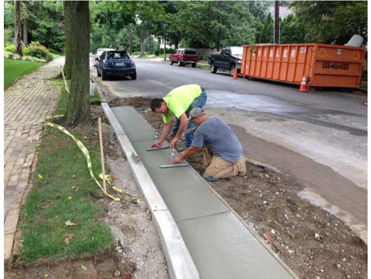
Constructing Curb & Gutter on Mountwell Avenue
