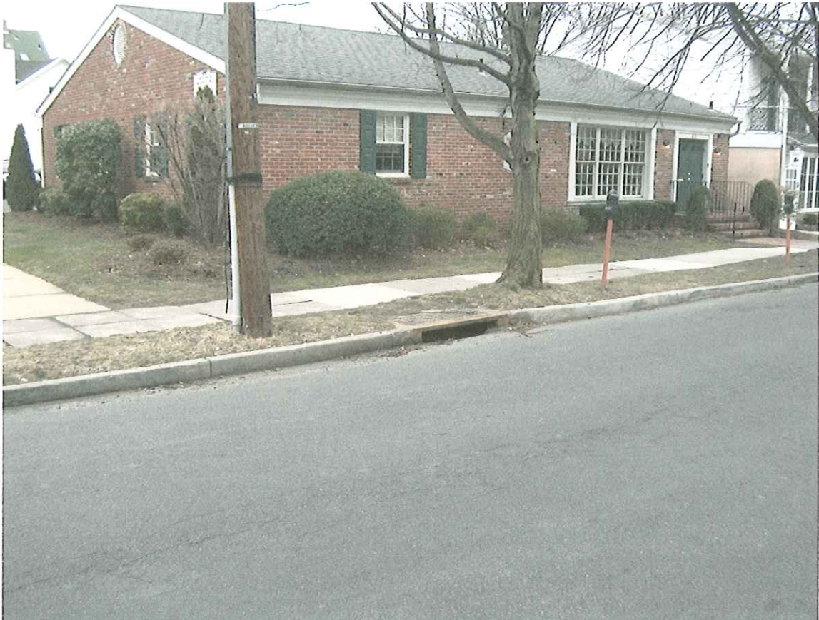
View of Existing Storm Sewer Inlet Near the Intersection with Wilkins Avenue
