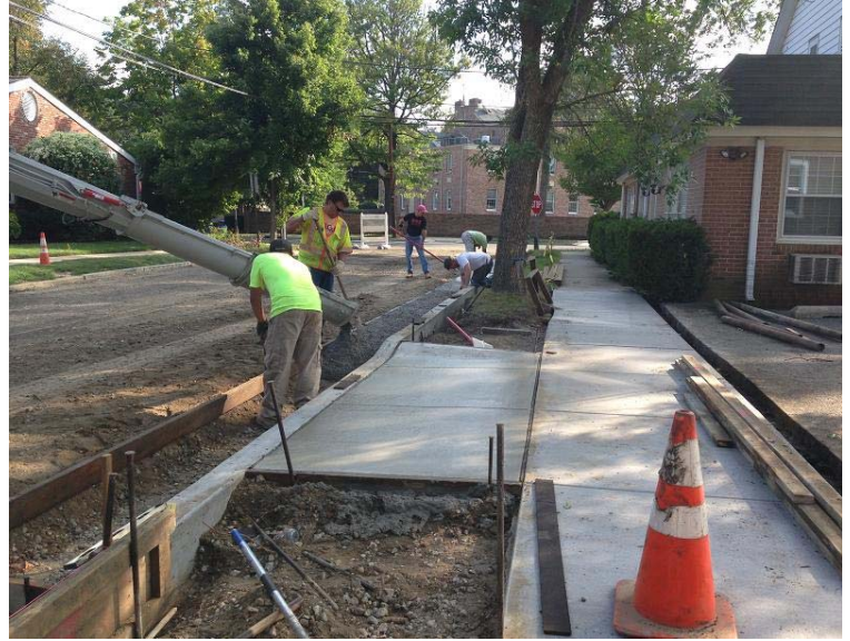
Constructing Curb & Gutter on Wilkins Avenue
