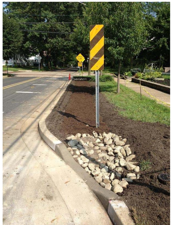
Rain Garden Constructed on Lincoln Avenue
