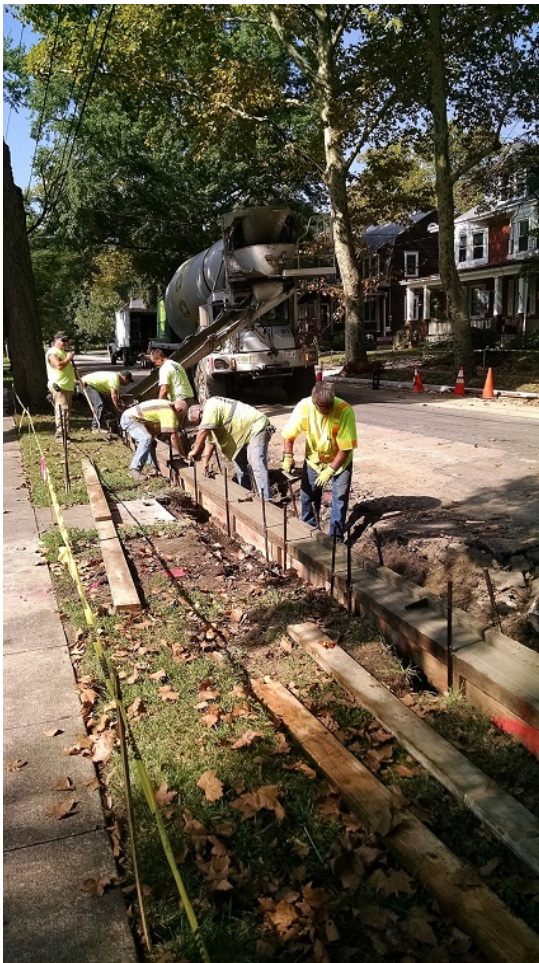
Pouring of Concrete Curb Along East Side of Mt. Vernon Avenue
