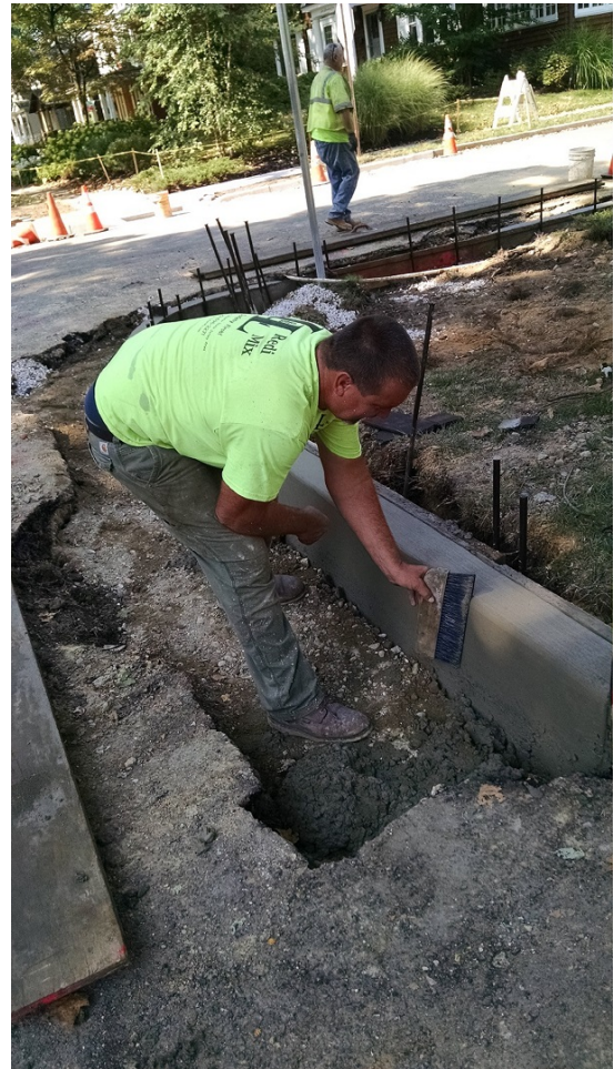
Finishing New Curb at Linden Avenue
