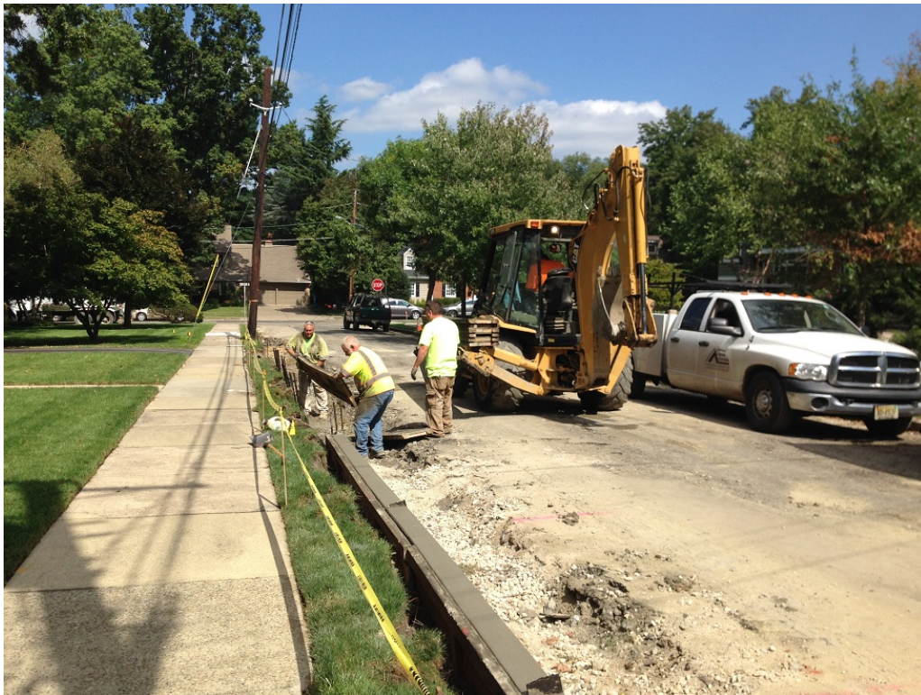
Construction of Concrete Curb Along West Side of Pomona Avenue
