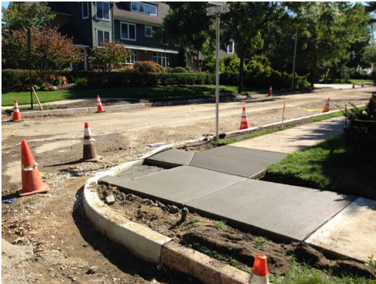
Newly Poured Concrete Sidewalk/ADA Ramp at Bellevue Avenue
