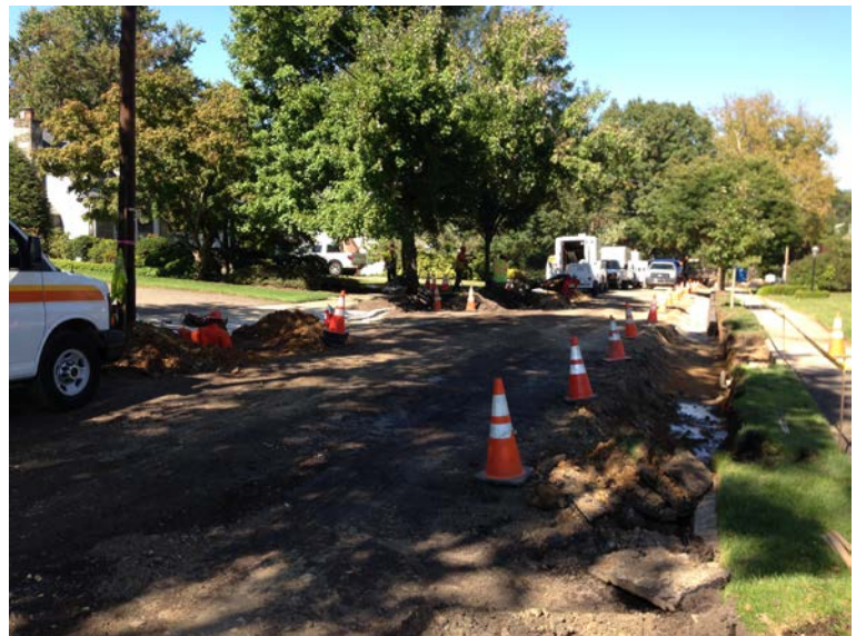
Installation of Gas Laterals at South End of Pomona Avenue
