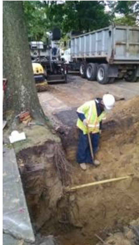
Contractor is excavating for the new utility installation.
