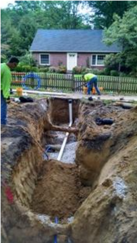
A new sanitary lateral is being installed.
