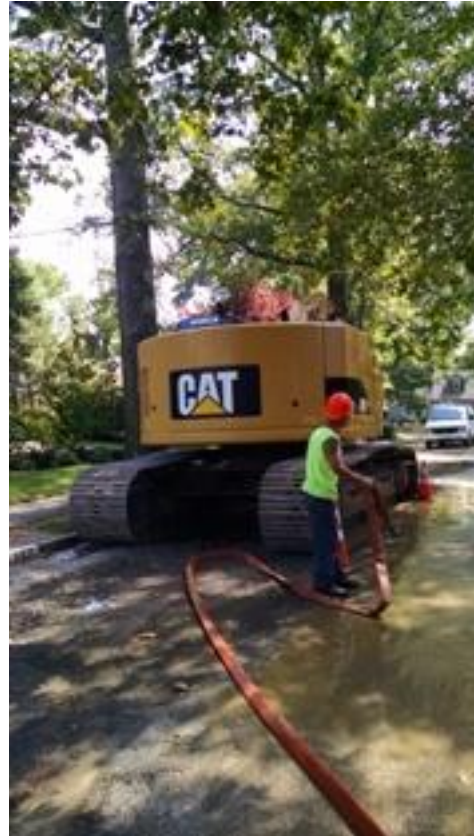
Roadway is wet down and swept for dust control.
