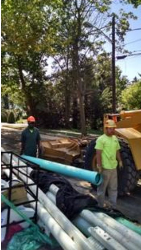
New sanitary sewer is being prepared for installation.
