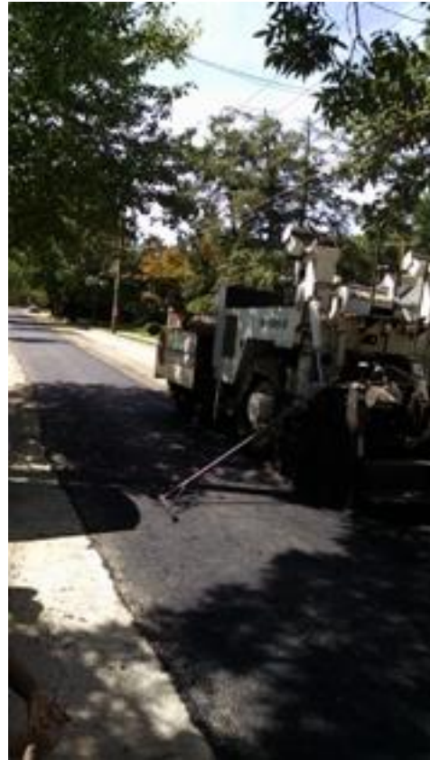
Utility trenches are temporarily paved.
