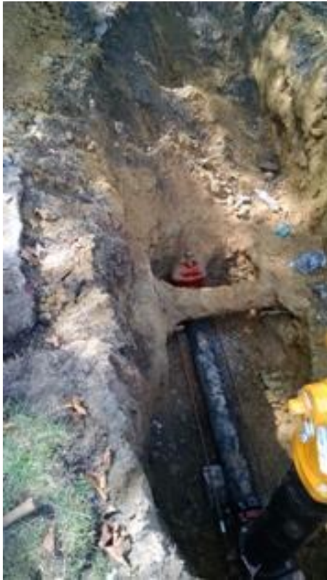
A new fire hydrant is installed.
