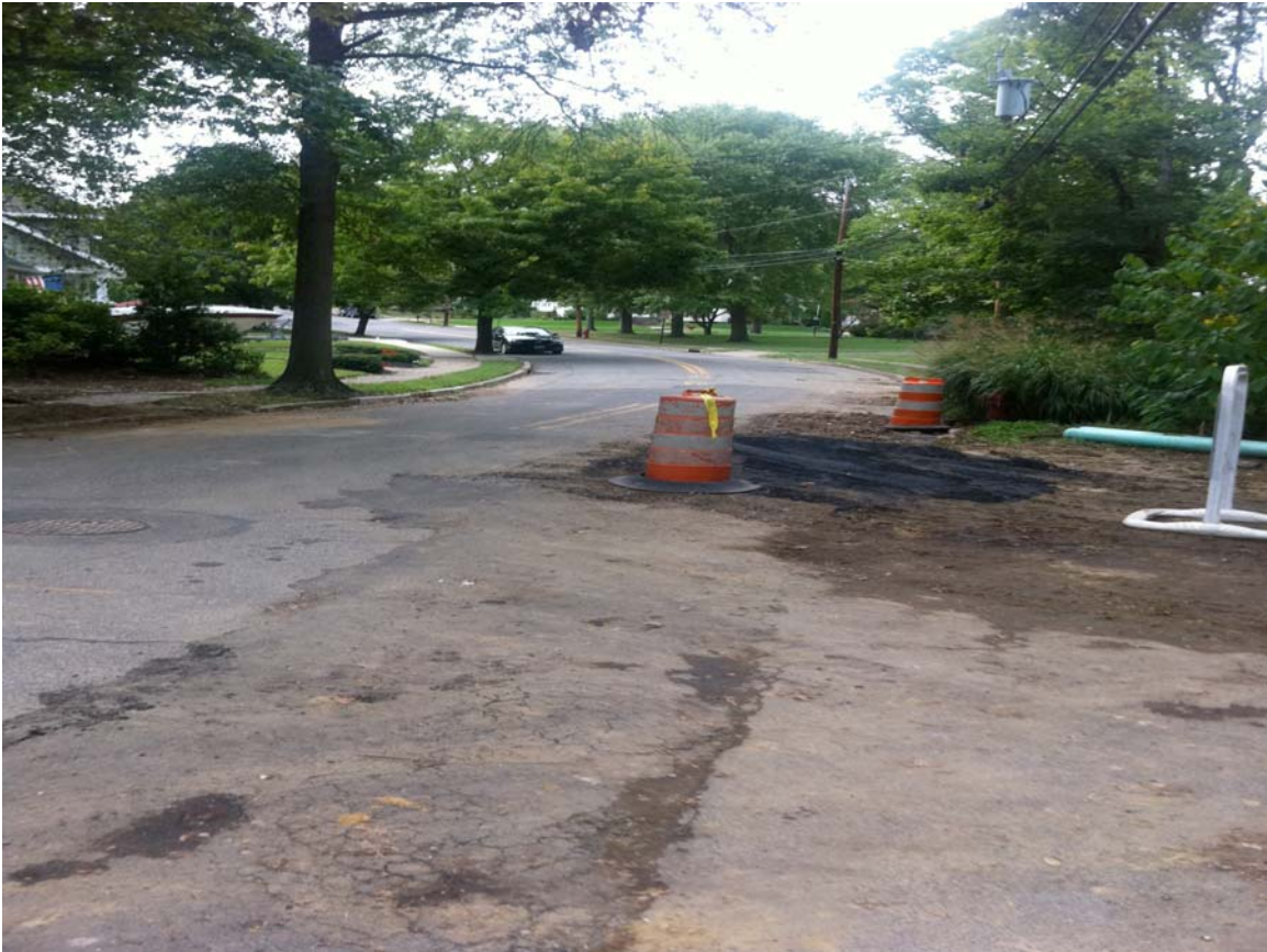
View of the Avondale Intersection on Wednesday Afternoon before the Storm
