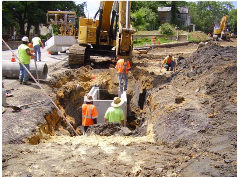
Installation of Inlet on Ellis Street @ Potter Street
