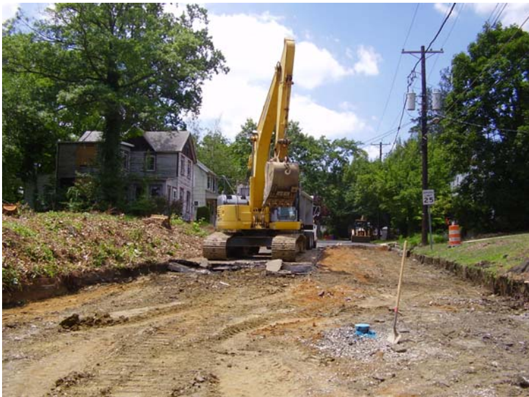
Removal of pavement on Potter Street
