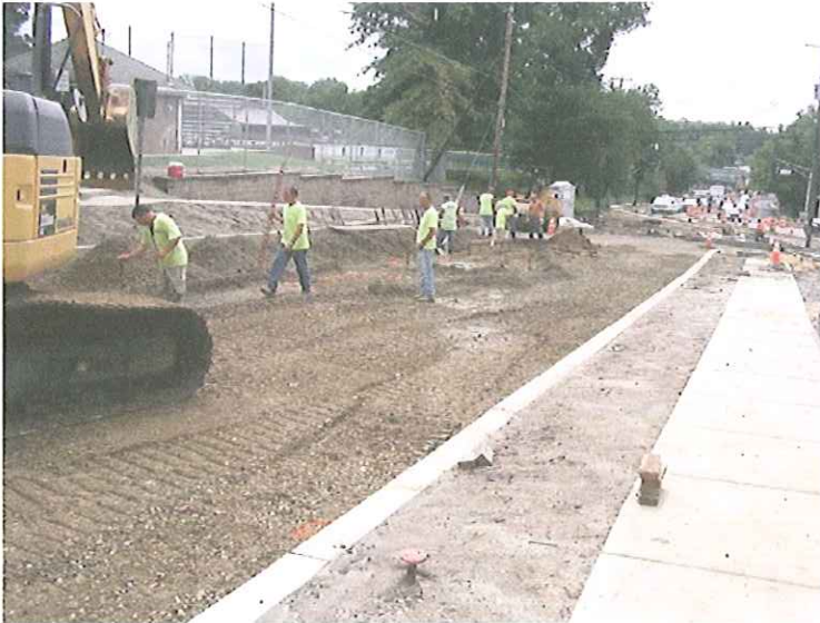
Placement of DGA Base Course On Potter Street
