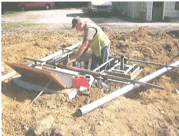
Construction of Traffic Signal Foundation at Kresson Road
