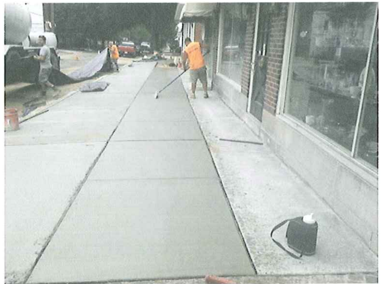
Sidewalk Construction At Kings Highway
