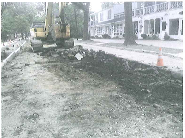
Roadway Excavation of Tanner Street
