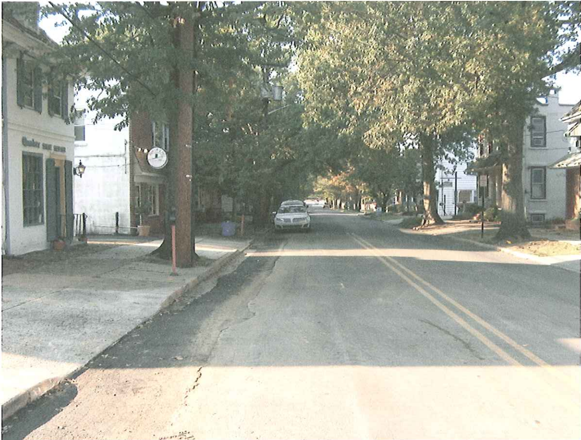
View of the New Water Main Trench Between Clement Street and Kings Highway East
