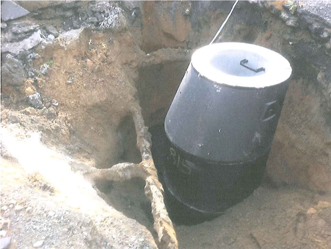
View of New Sanitary Sewer Manhole at Clement Street
