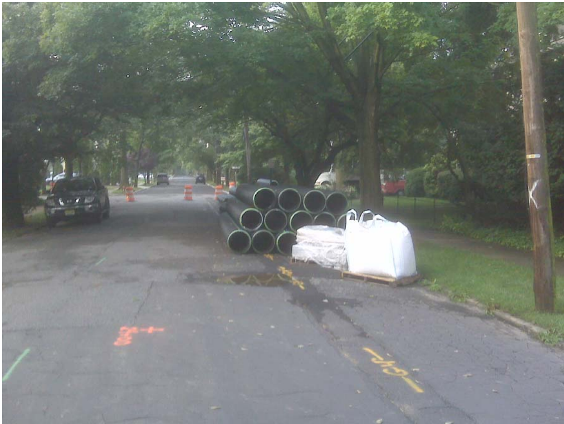
18" Diameter Plastic Storm Sewer Pipe Waiting to be Installed
