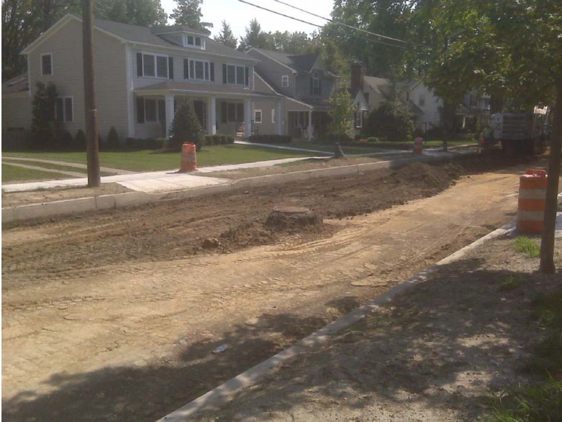
The 500 Block as the Contractor is Excavating for the New Roadway
