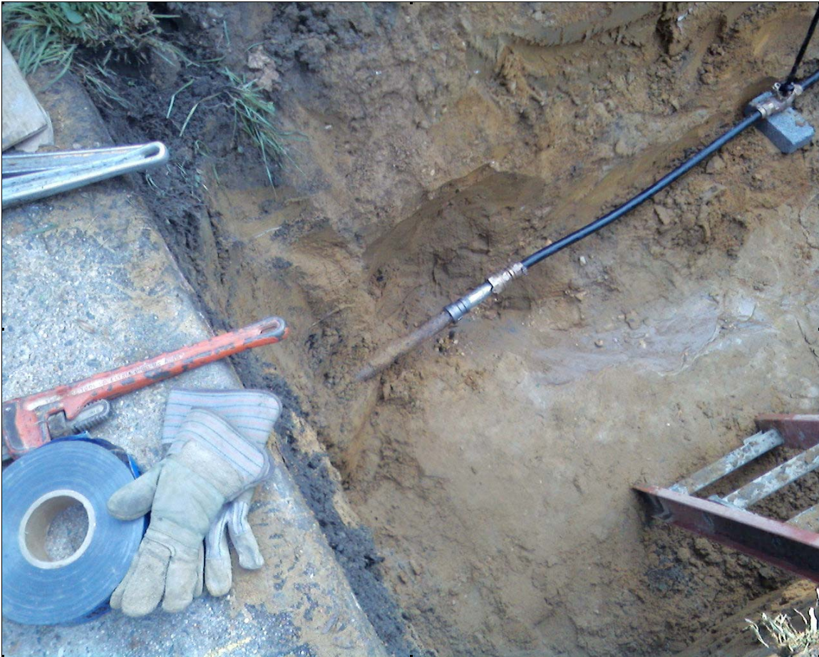
A Recently Completed Water Service Replacement
