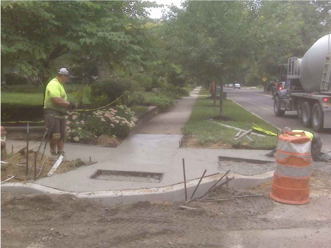
The Concrete Crew Pouring a New Handicap Ramp
