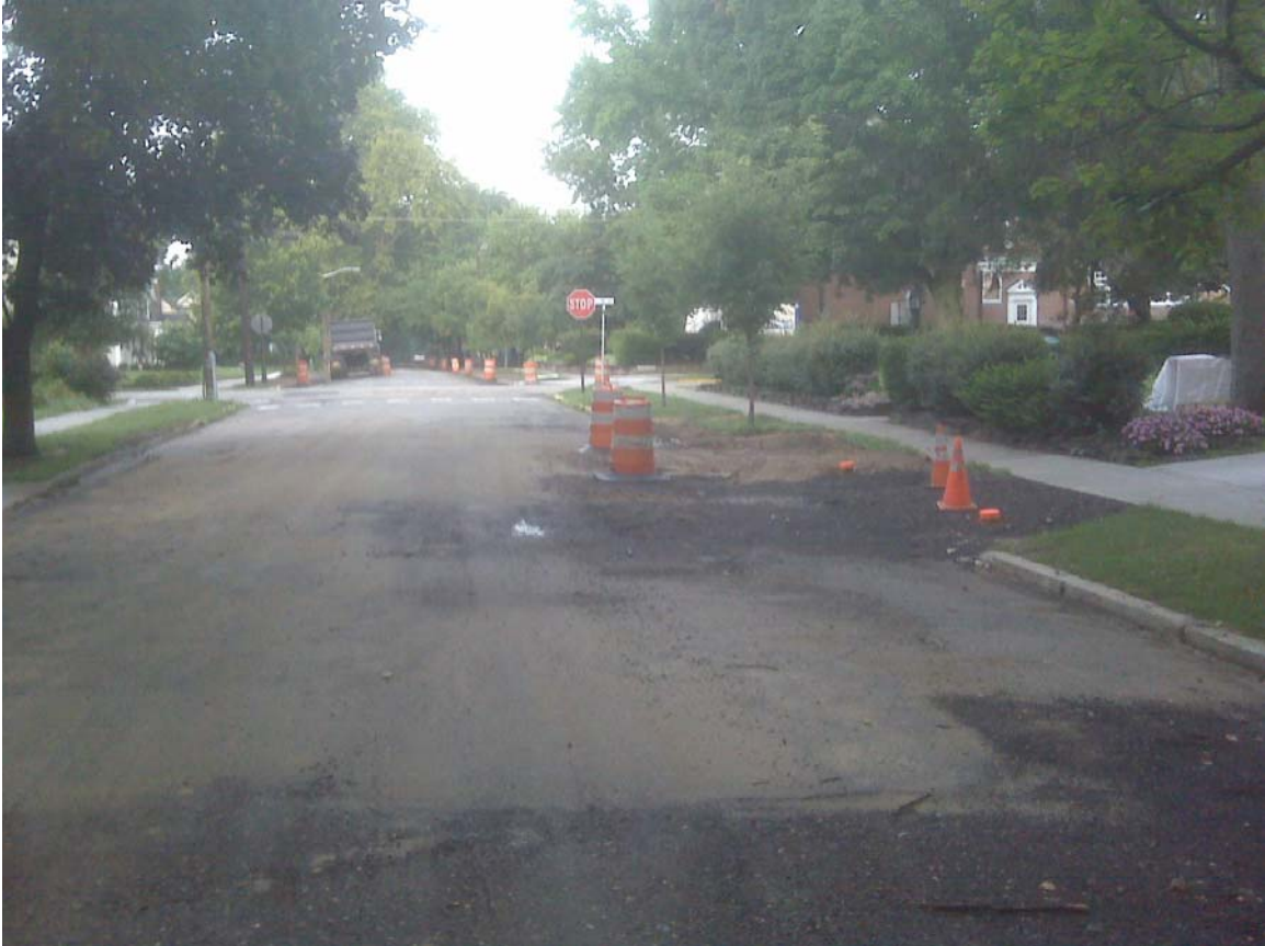
The Location of the New Sanitary Sewer Manhole
