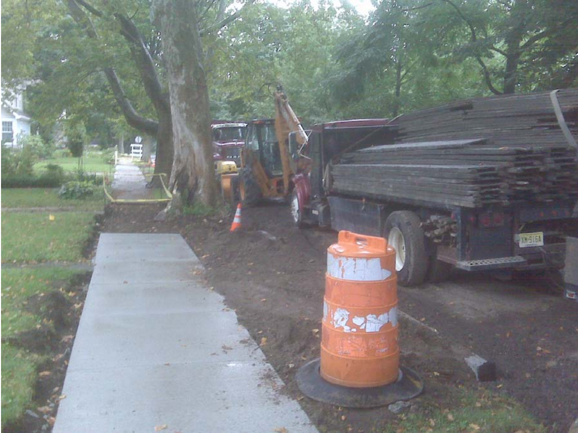
Missing Sidewalk and Driveway Apron at 518 Redman Avenue
