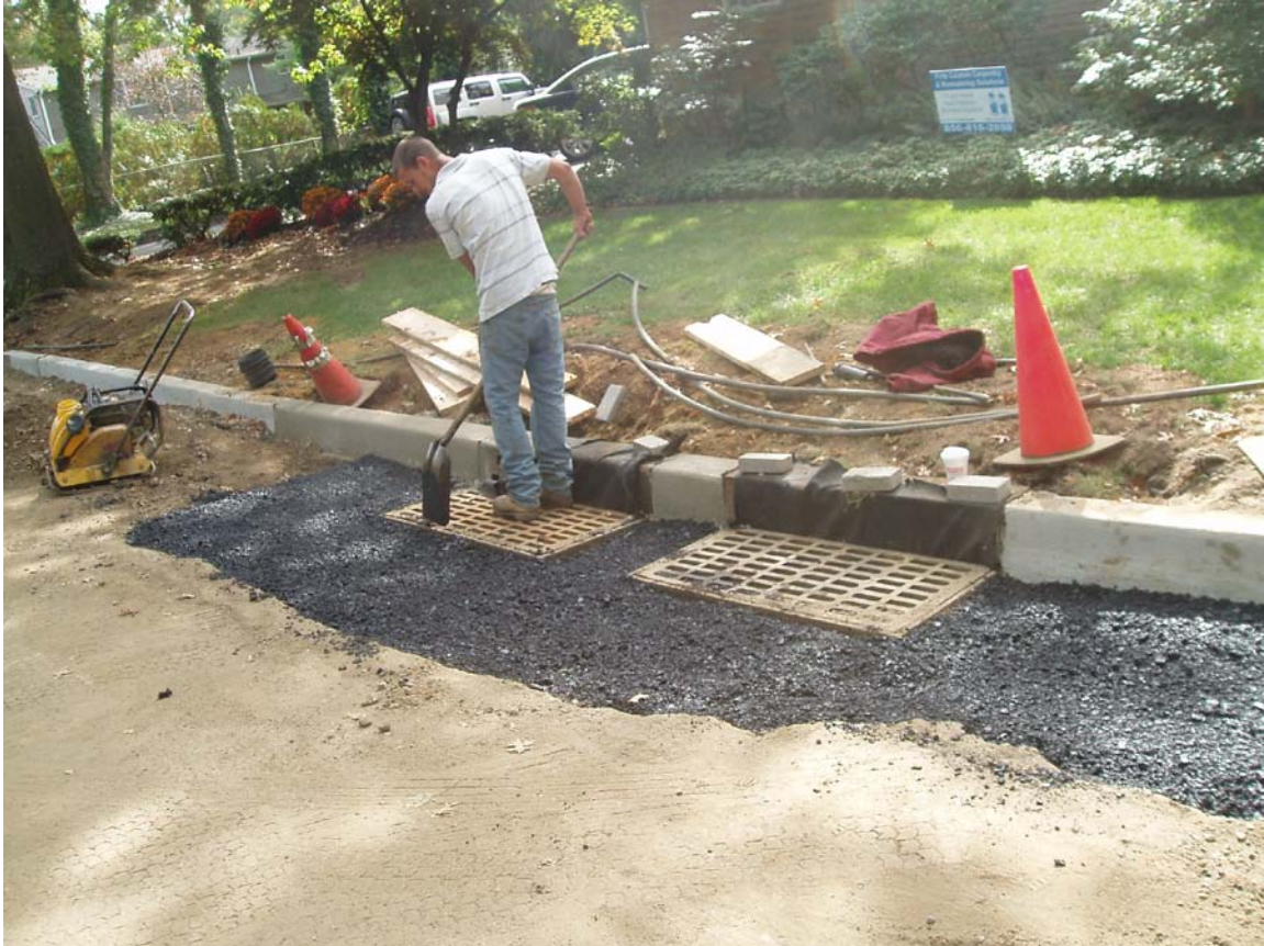
View of Stormwater Inlet Repairs
