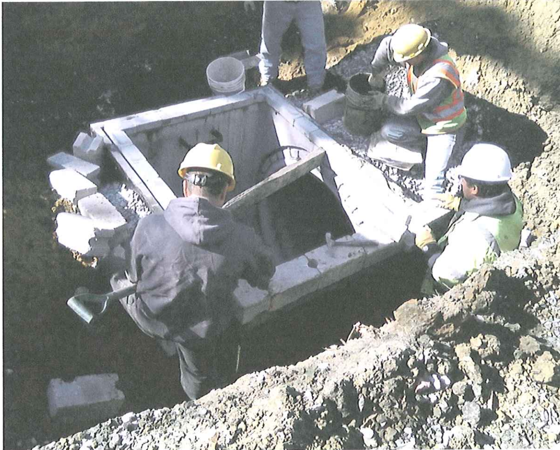
View of the Installation of a New Storm Sewer Inlet Structure at the Clement Street Intersection
